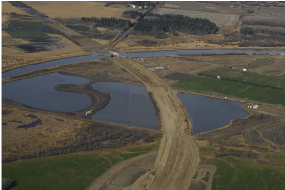
Aerial view of the West Regional Road crossing Sturgeon River
