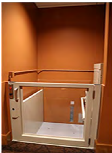
Lift to studios
